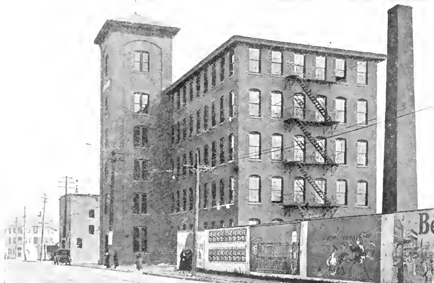
CUSHMAN & HEBERT FACTORY, RIVER STREET
